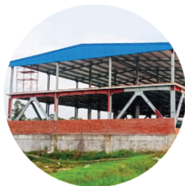
STEEL SHED WITH MEZZANINE FLOOR
