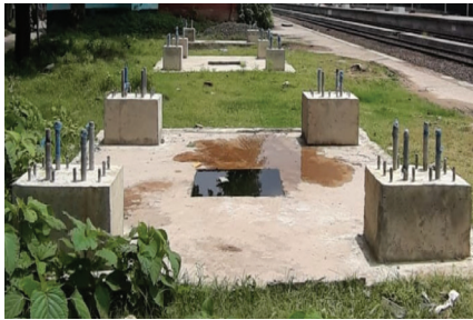
FOOTING & SHORT COLUMNS
