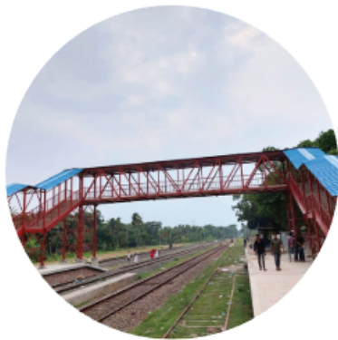
FOOT OVER BRIDGE
